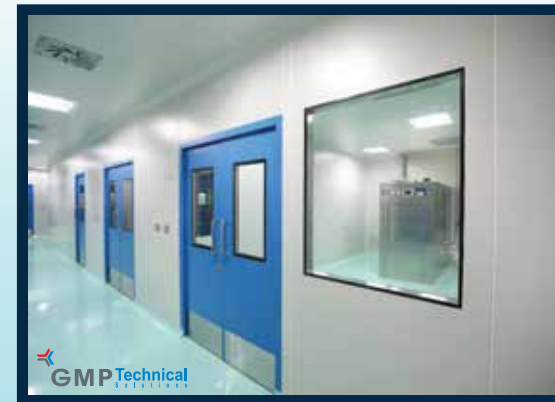
Clean Room Partitions, Walls, Ceiling & Doors
